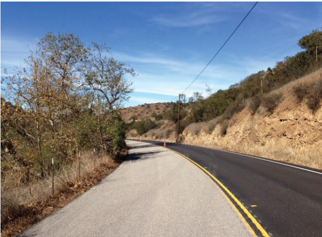
Friction Course – Finished Installation
