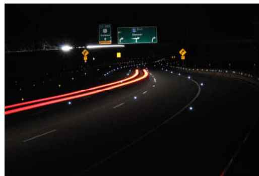
EB I-70 at US-6, Jefferson County
